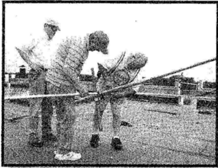
Joseph Lowenthal, WA4OVO, of Memphis; Frank McDowell, KA4SJM (NNNØANX), Bartlett, TN; and Alexander Hilliard, W4GMM (AFA2FL), Memphis install the rooftop 14-MHz beam antenna at WUG-231, the U.S. Army Corps of Engineers station near Memphis. Photo by James Pogue KH2AR.
