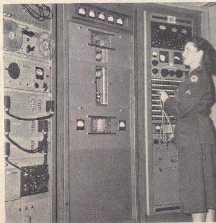
Cpl. Laffer patches a keying line from the local transmitter (center bank) into an adjoining studio at headquarters station.
