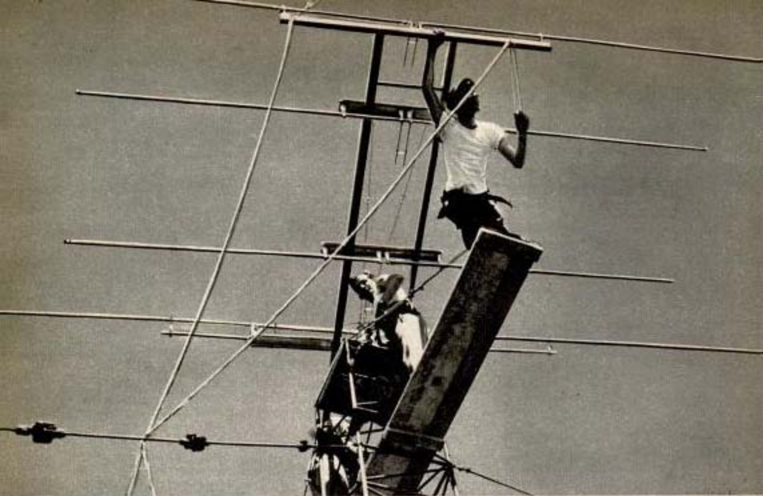
Atop the Pentagon Building, Air Force personnel erect an antenna for broadcasts beamed by MARS station K4AF
